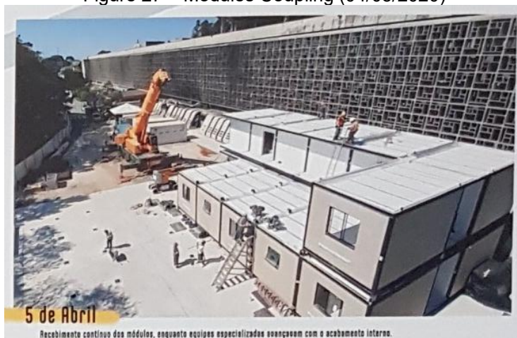
Figure 27 – Modules Coupling (04/05/2020)
