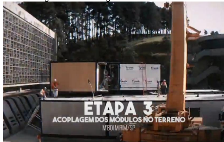
Figure 26 – Docking of the modules on site
